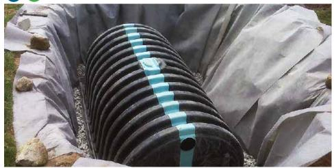
A dry well is a subsurface stormwater facility consisting of either a structural chamber or stone filled excavation that is used to collect and temporarily store stormwater runoff from rooftops. The dry well inflow is connected by roof leaders. The sides and top of the dry well are completely lined with filter fabric to avoid fines clogging the system.
