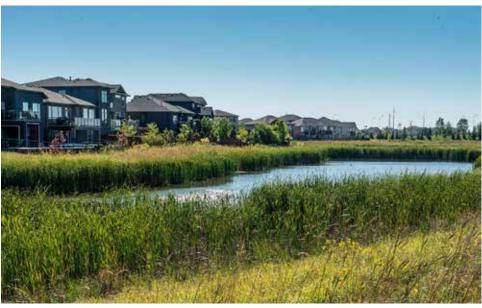
A wet pond is a permanent pool where stormwater is captured and regulated by an elevated outlet structure. Native vegetation should be used to provide a permanent buffer around the pool. Water from the pond should be used for irrigation or some other beneficial use.
