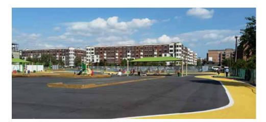
Existing conditions at the Northwest Resiliency Park site in the City of Hoboken, NJ. The site is a brownfield site contaminated by former industrial uses. The temporary pop-up park shown is constructed on an asphalt cap. No stormwater management exists.
