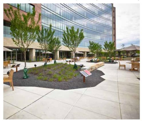
through sheet flow and by using surface swales rather than underground piping, construction costs were reduced. Through this green infrastructure approach, the first flush of runoff has a greater opportunity to be completely retained on site and infiltrated to groundwater.
