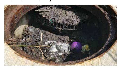
The sediment filter trap shown in the image has done its intended job and kept a large amount of sediment, trash, and debris out of the downstream system. It needs to be cleaned out in order to maintain its functionality. Image Credit: E&LP, 2020
