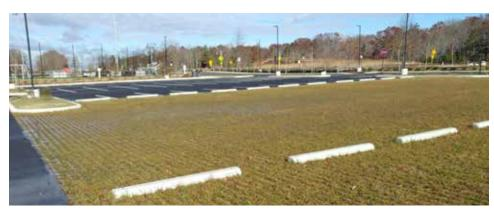
Pervious pavement is a surface that allows water to infiltrate into the ground below. Pervious pavement materials can include asphalt, concrete, interlocking concrete pavers, gravel, and resin-bonded materials such as recycled rubber, mulch, and glass. These surface courses are installed over a supporting base of crushed stone that helps to store and infiltrate stormwater.
