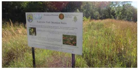
Extended detention basins are surface depressions that temporarily store stormwater runoff. The slower drain time allows sediment to settle to the basin bottom before water discharges. The amount of water quality treatment is dependent upon the detention time.
