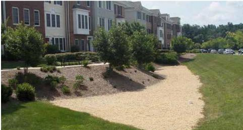
A sand filter at the base of a planted slope. Image Credit: Montgomery County, MD, 2018
