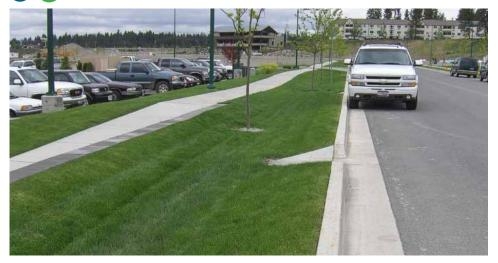
A grass swale is a long, narrow grassy channel used to convey stormwater to a downstream green infrastructure practice or storm drain. Grass is typically kept to a height of about three to six inches to slow down the runoff and allow any debris or sediment to settle out without interfering with the direction of flow. Depending on site conditions, additional features such as check dams and underdrains may be required to comply with New Jersey Soil Erosion and Sediment Control Standards.
