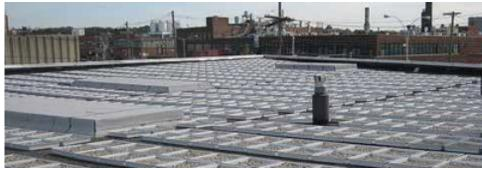
Blue roofs are non-vegetated systems that hold stormwater. They can be designed as modular trays with loose stones, specialized permeable pavers, or just a waterproof membrane.
